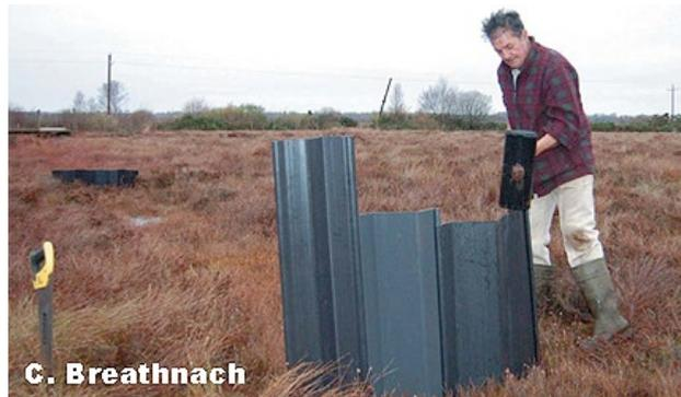
Plate 8-40: Plastic piling being installed within IPCC bog
